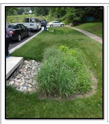
Throughout the Breewood Manor community, green street landscaping was incorporated into the restoration plan. Hot, polluted runoff from the roads and other hard surfaces has been diverted into specially designed rain gardens where the runoff will be cleansed and cooled off.
