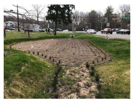
looked dormant, soon nine species of plants will fill the mulched area. The mulch and soil root zone help absorb stormwater runoff and, using a process called phytoremediation, break down pollutants such as oil on roadways. The stormwater runoff collected from the surrounding roads and other hard surfaces when it rains percolates through the special bioretention soil.
